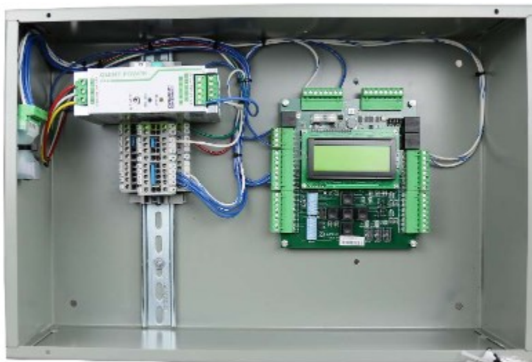
Figure 3: Car Top Controller
