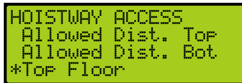
Figure 399: HOISTWAY ACCESS – Top Floor
