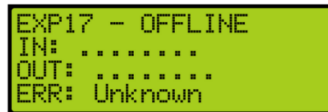
Figure 633: Inactive Expansion Board Status
