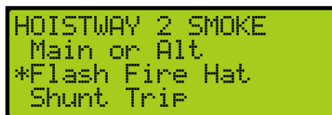
Figure 600: HOISTWAY 2 SMOKE Menu – Flash Fire Hat
