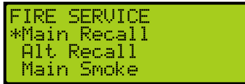
Figure 546: FIRE SERVICE Menu – Main Recall
