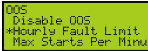
Figure 448: OOS Menu – Hourly Fault Limit
