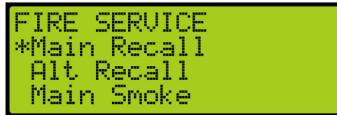
Figure 462: FIRE SERVICE Menu – Main Recall
