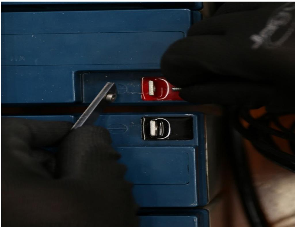
*Figure 10: Bus Bar Connecting Both Sides of Batteries*
